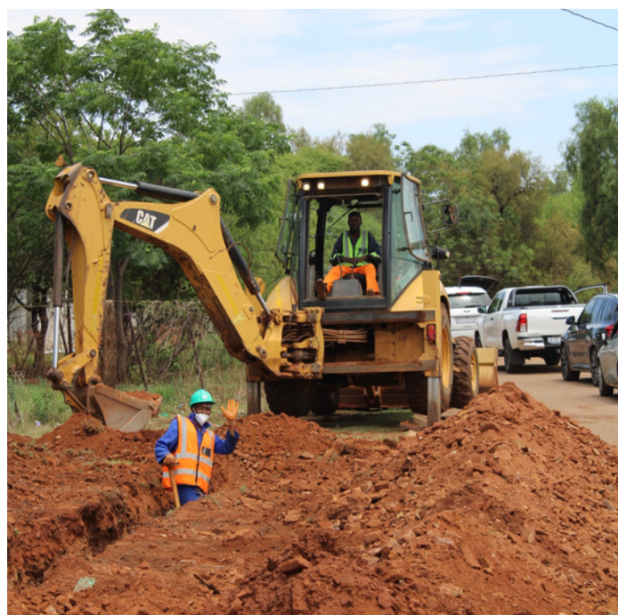
Magalies Water's appointed main contractor has dug trenches, where a new pipeline running through Dinonaka Village will be installed, to avail water to high-lying areas, which have been struggling to access piped water
